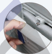
Filter mat replacement method
